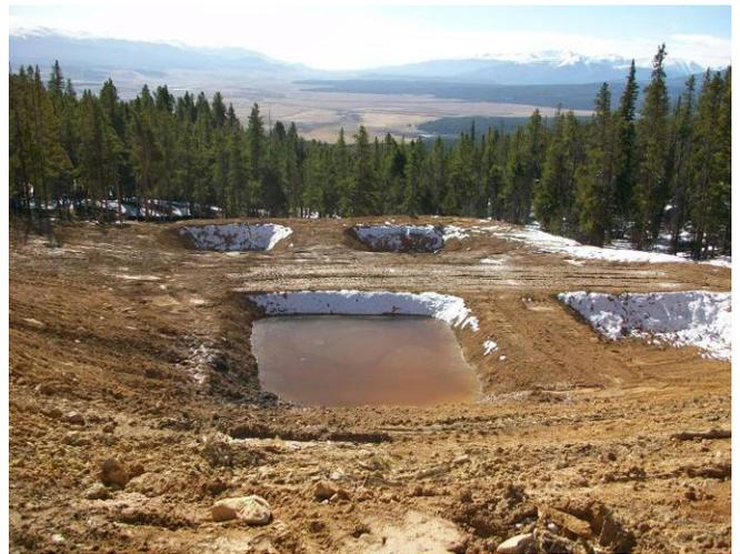
*At the completion of the removal of the mine waste pile and the construction of the repository, future SRB cells were excavated. These cells will likely remain empty and inactive until the passage of federal Good Samaritan legislation.*
